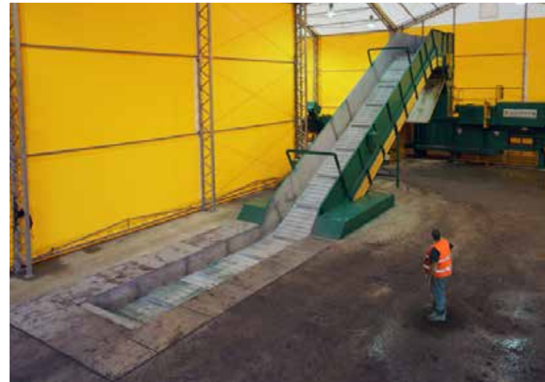
LOADING SECTION OUT OF PIT
