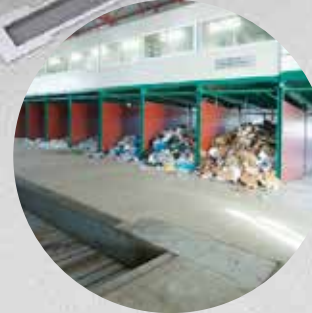
RECYCLABLE MATERIAL STORAGE BUNKER
