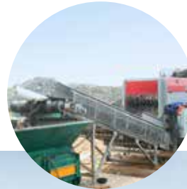
SCREENED WASTE COLLECTION BELT
